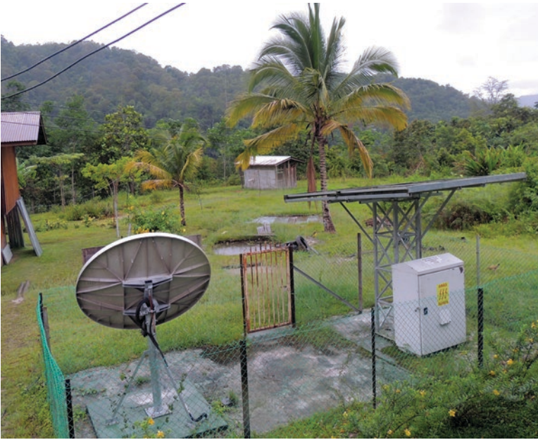
Fig. 26.4 A village micro-grid energy and telecommunications system in the Crocker Highlands of Sabah, Malaysian Borneo. The system serves a community of 200 and provides household energy services, telecommunications, and a satellite communications (dish shown), water pumping for fish ponds (seen in the center), and refrigeration. The supply includes micro-hydropower and solar generation (one small panel is shown here; others are distributed on building rooftops). (Photo credit: Daniel M. Kammen)
