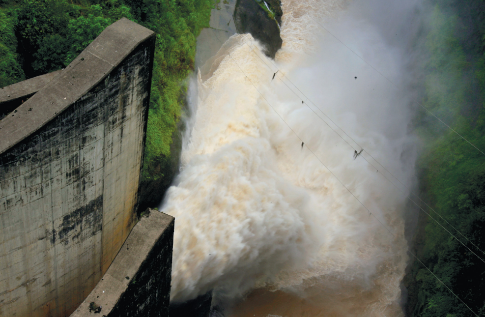
Facilities like Costa Rica's Cachi Dam provide power, flood control, and recreation, but can also carry high social and environmental costs.
