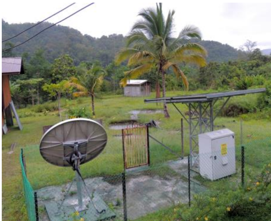
Figure 4: A village micro-grid energy and telecommunications system in the Crocker Highlands of Sabah, Malaysian Borneo. The system serves a community of two hundred, and provides household energy services, telecoms and satellite (dish shown), water pumping for fish ponds (seen at center) and for refrigeration. The supply includes micro-hydro and solar generation (one small panel shown here, others are distributed on building rooftops). Photo credit: Daniel M. Kammen.
