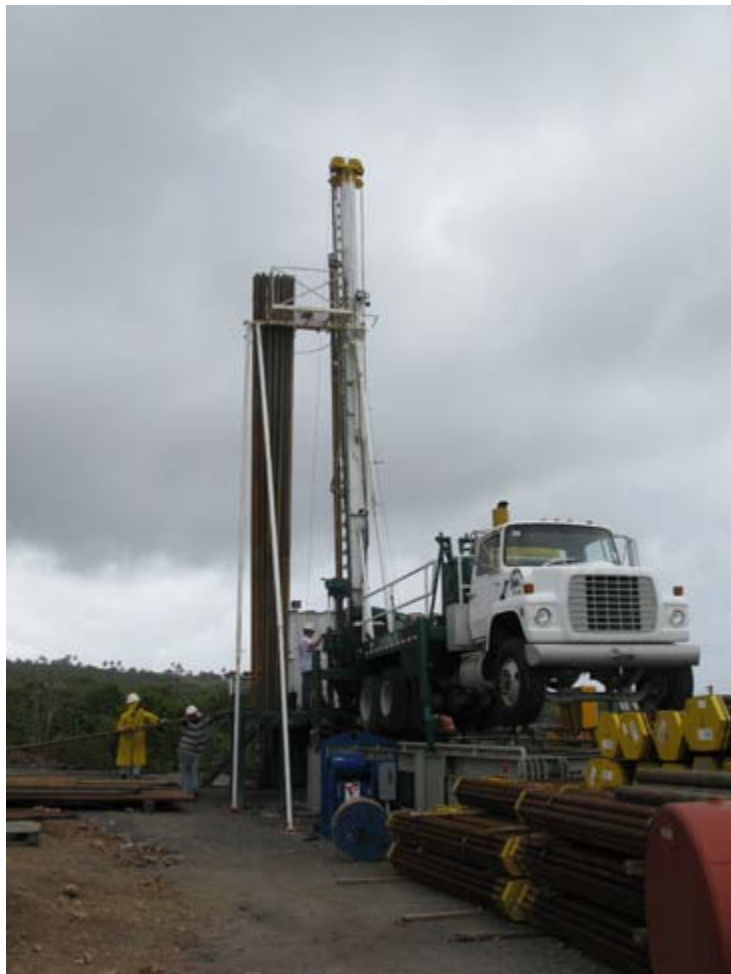
Geothermal slim-hole drilling, Nevis (St. Kitts and Nevis)
