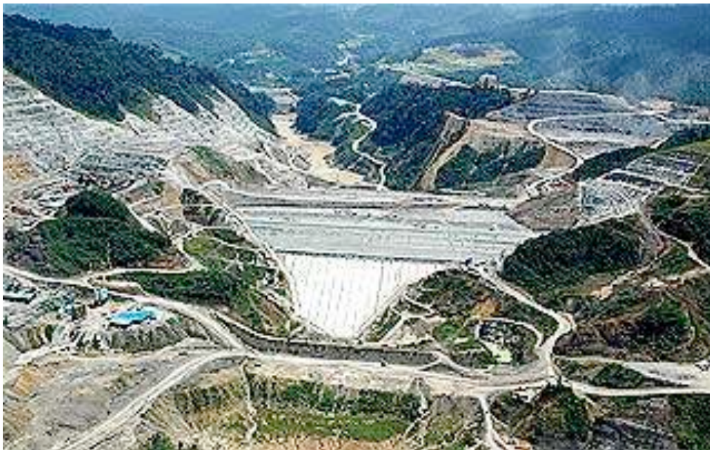
Figure 2-3a: The Bakun Dam Construction Site 88
