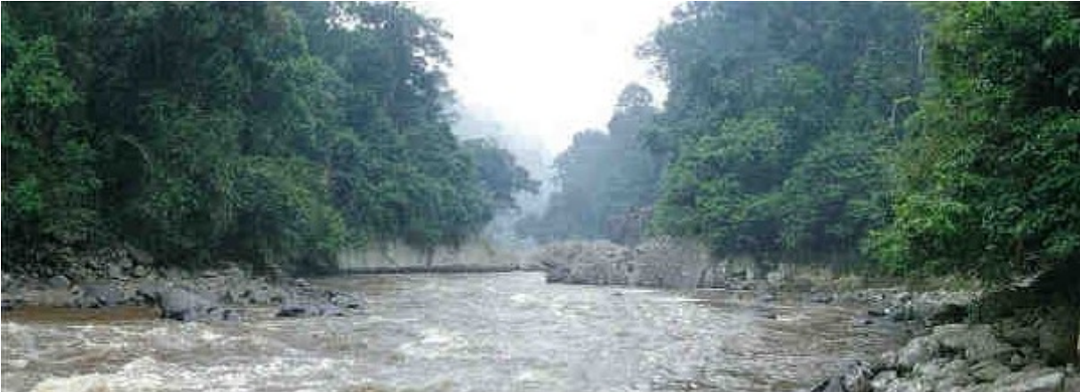
Figure 2-3: Upper Padas 150 MW Proposed Dam Site 87
