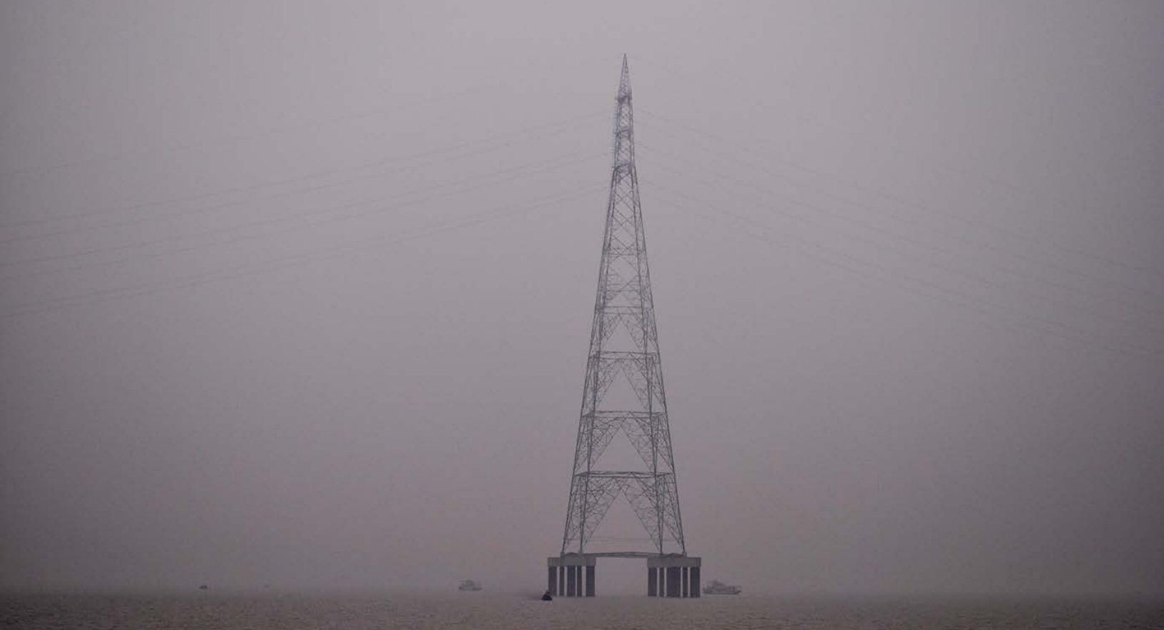
Off-shore transmission line connecting the Sundarbans Islands to the West Bengal central electric grid
